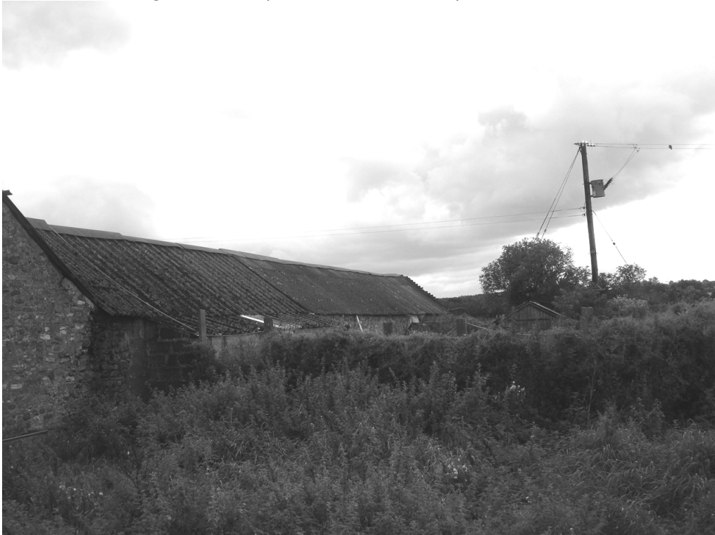
Plate 2: Existing structure (Northern Elevation)
