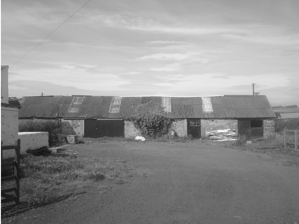
Plate 1: Existing structure (Eastern elevation)
