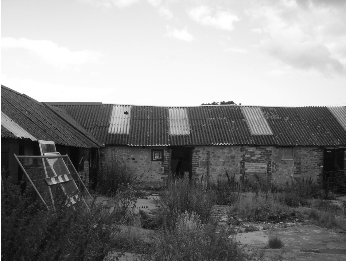
Plate 5: Existing structure (Western elevation)
